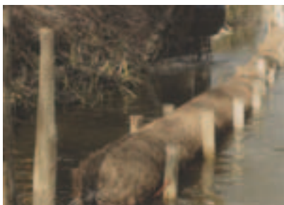
Coir rolls protecting the river bank
