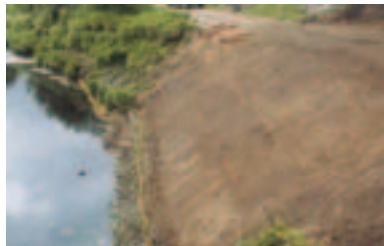
Regraded bank before vegetative establishment
